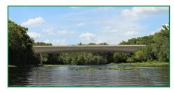
includes a parallel, non-tolled, service road for local travel, and a new, much higher bridge with a slightly arched design and other aesthetics over the Wekiva River.
